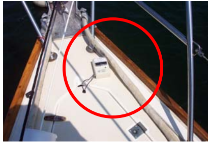
High moisture between bow rail mounts starboard.
